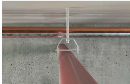
Sprinkler pipe installation
