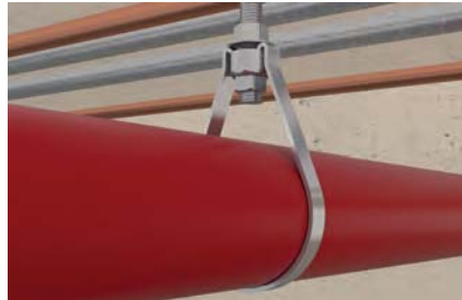
Sprinkler pipe installation
