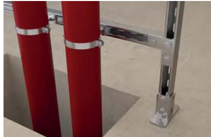
Waste water pipe
