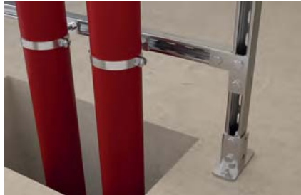
Waste water pipe
